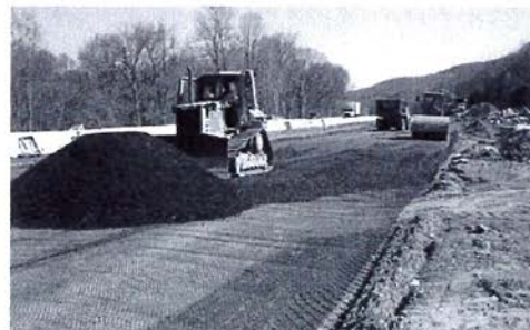
IMAGE 9B: Spreading aggregate fill over Tensar Geogrid.
