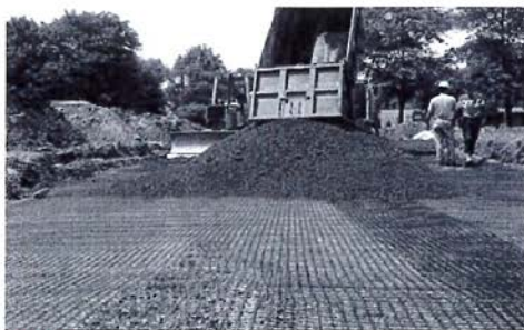
IMAGE 9A: End dumping aggregate fill on top of Tensar Geogrid over soft subgrade.
