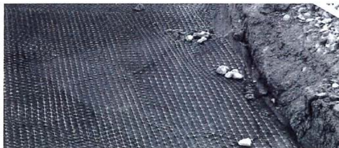
IMAGE 7: Anchoring geogrid with piles of aggregate.
