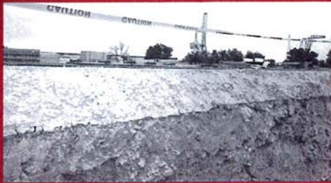
IMAGE 13: A backhoe excavation through Tensar Geogrid.
