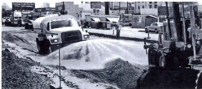
IMAGE 10: Moistening the fill before compaction.
