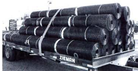
IMAGE 2: Storing the Tensar Geogrid rolls horizontally.
