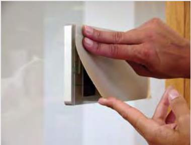
GLASS (G) Aggressive double-back tape applied to the sign backer plate. Includes mask for the back side of the glass.
