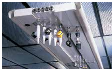
Overhead service enclosure with quick connect fittings
