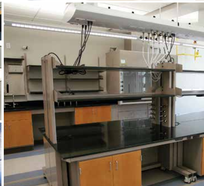
Overhead service enclosure with quick connect fittings
