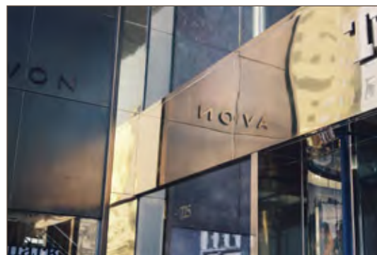
Figure 3.1B. The specular or mirror finish on this facade reflects the colors and images of its environment.
