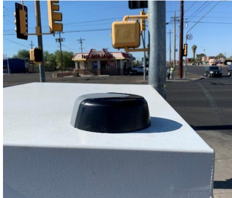
Figure 19: Antenna mounted to top of cabinet
