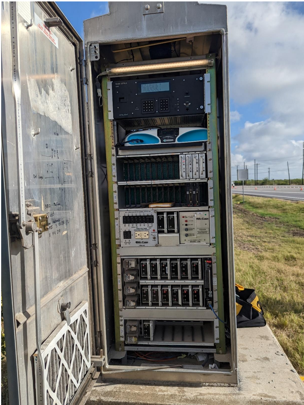
Figure 37: Front view of 332 cabinet after installation.
