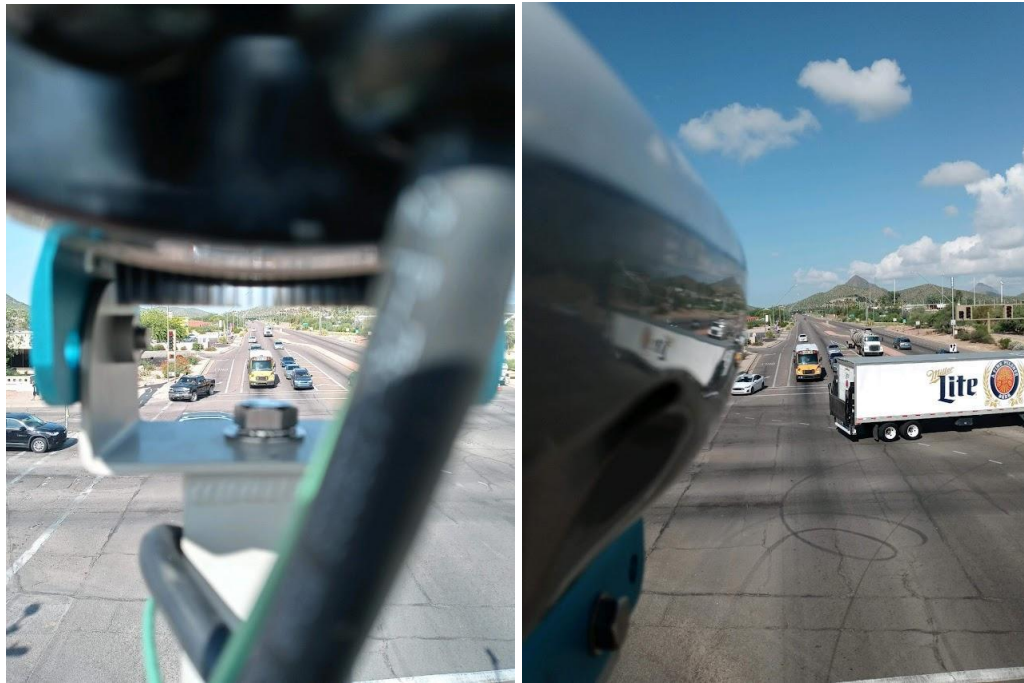
Figure 33: Sensor Unit initial aiming guidance
