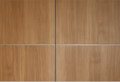
Outserts are slightly proud of the frame and create a uniform look for the surface material while creating a subtle reveal.
