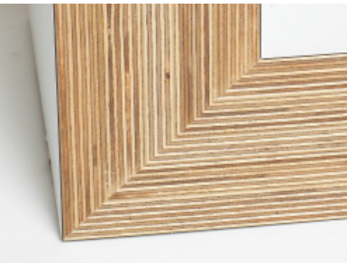
Base miter detail of exposed baltic birch ply
